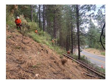
Crews with P31 Enterprises Inc. performed wood management, removing any trees with potential to strike the road or that could become fuel for fire near the road, then clearing brush and the debris from tree removals.
